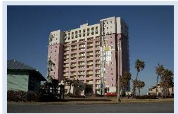
A hotel in Pensacola, Florida damaged by Hurricane Ivan in 2004.
